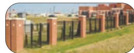
Shown above is another stretch of the fenceline. Unseen are the massive footers which anchor the fence. These were backfilled with dirt and are not visible. (Hercules Fence photos)
